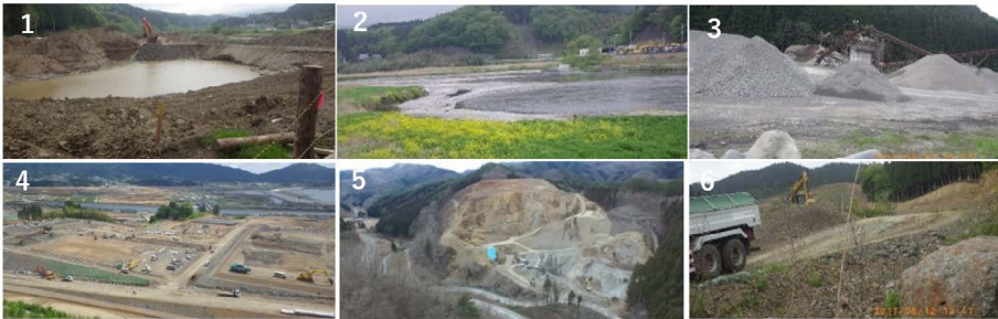
Extraction of gravels and soil for reconstruction works in Rikuzentakata City 1: Gravel extraction site (former rice paddy) 2: Site after extracting river bed gravels (Kesen River) 3: Extracted gravels piled up (Kesen River) 4: Land is raised using soil from mountains to develop residential areas (Sanriku Motorway running in front) 5: Mt. Iimori quarry site 6: Soil extraction site
